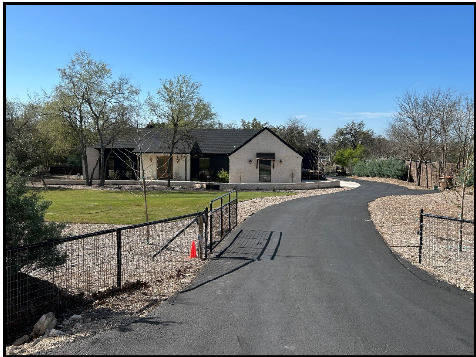
Figure 4: Rock landscaping beds reduce structure loss risk by breaking up horizontal fuel continuity between the structure and fuels while also reducing risk of landscape plants igniting.
