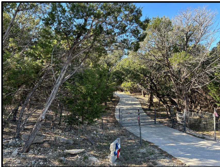
Figure 5: Dense and overhanging vegetation can limit the access of emergency vehicles to the structure. These trees should be pruned to allow vertical access of at least 13.5 feet.
